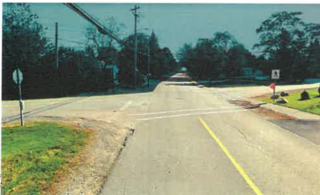
Crosswalk with markings, flags, and signage
