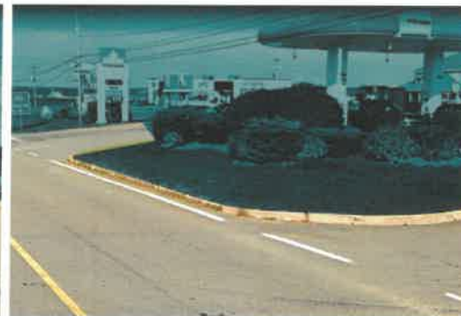
Crosswalk and sidewalk missing
