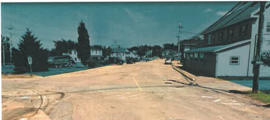
Crosswalk with faded marking and no signage
