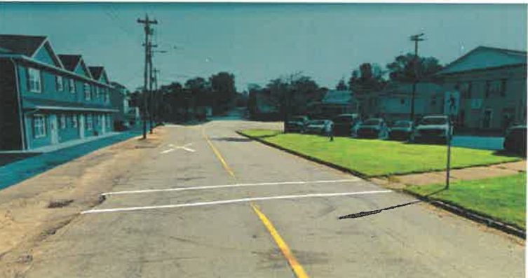
Narrow crosswalk with signage on one side, and no sidewalk on either sides
