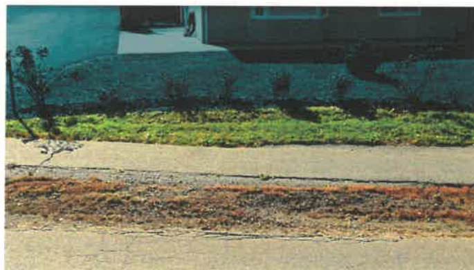
Asphalt sidewalk with signs of wear, no curb, and little buffer from road
