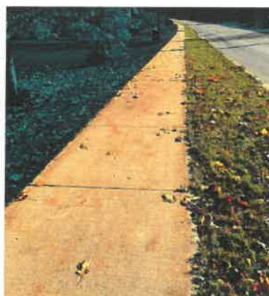
Concrete paving with even surface
