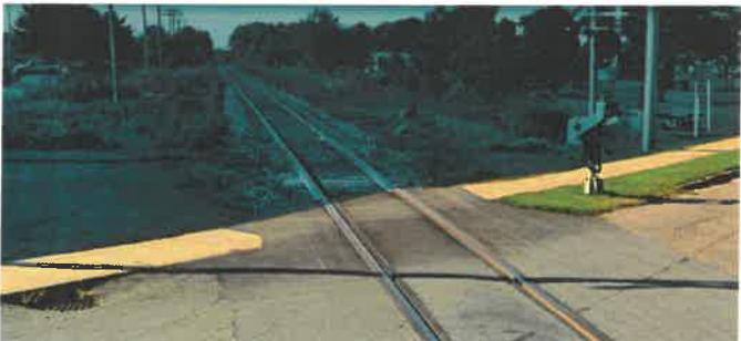
Hazard prone crossing with no curbs on one side of the sidewalk
