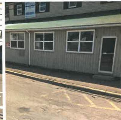
Concrete sidewalk with curb in small section of the segment
