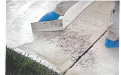
Concrete overlay/ Resurfacing
