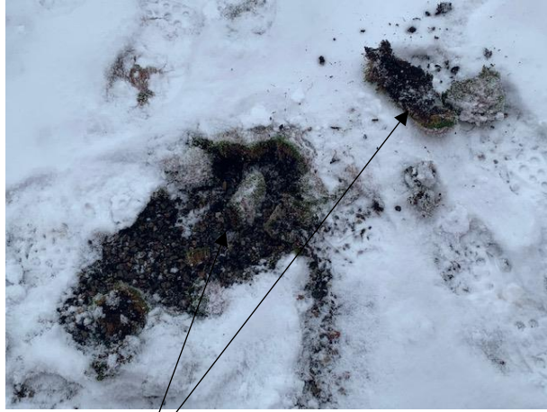
moss growth covered several areas
