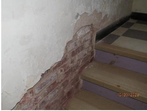
Stair to basement
