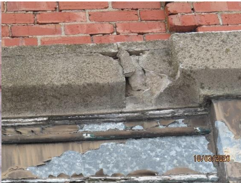
open masonry, water infiltration
