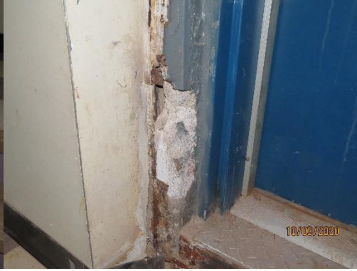
Exterior door to south stairs to basement
