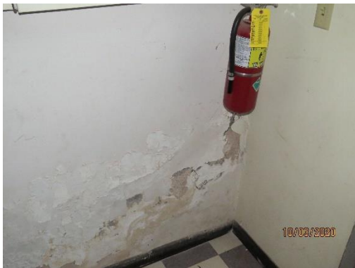
Near south door
