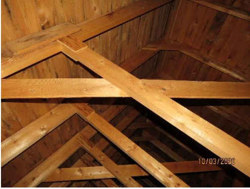
Attic space- no visible leaks
