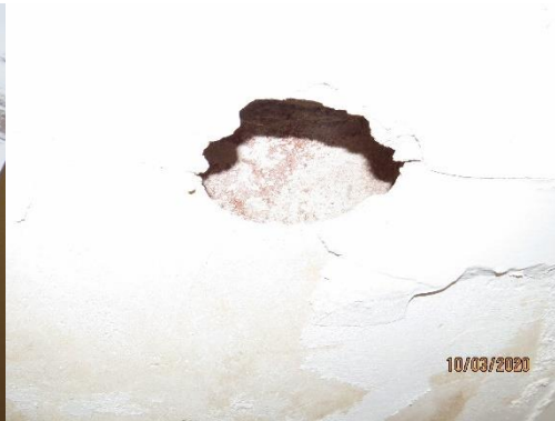
Hole in drywall, north wall upper floor No insulation, exterior masonry visible
