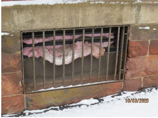
At boiler room
