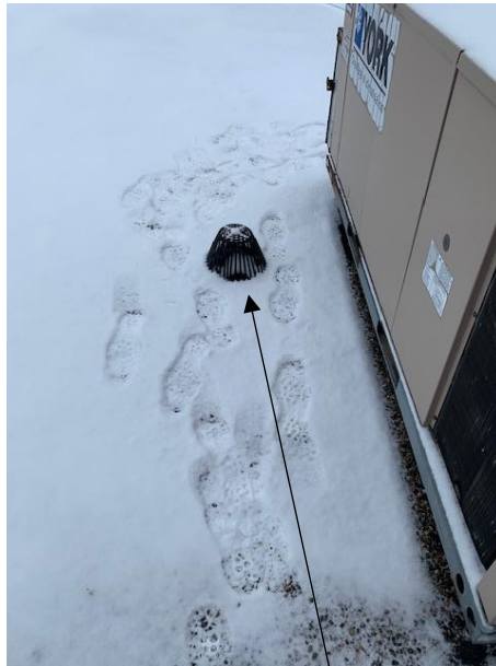
1 roof drain found near HVAC unit
