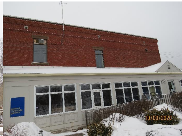
Former art gallery extension to Town Hall building
