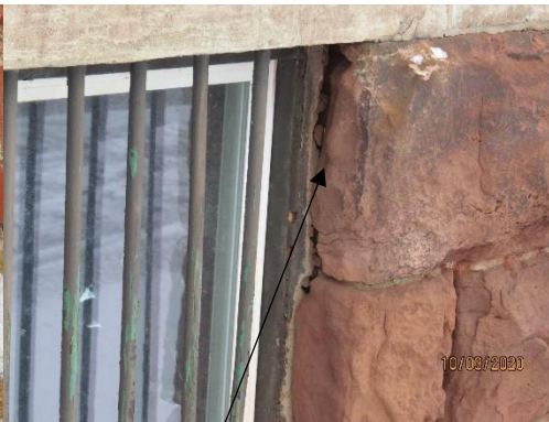
open masonry, water infiltration
