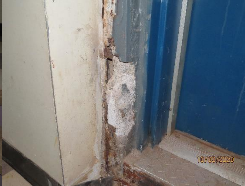
Exterior door to south stairs to basement
