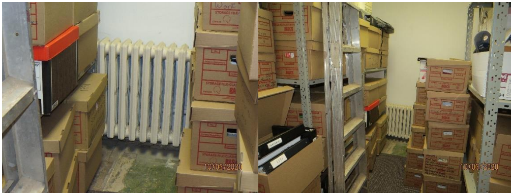
Records storage fire hazard
