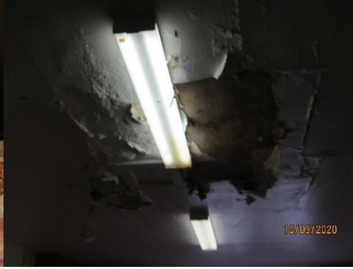
Interior upper floor water leaks and mould
