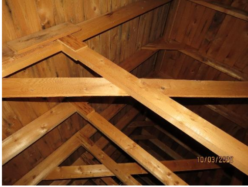
Attic space- no visible leaks
