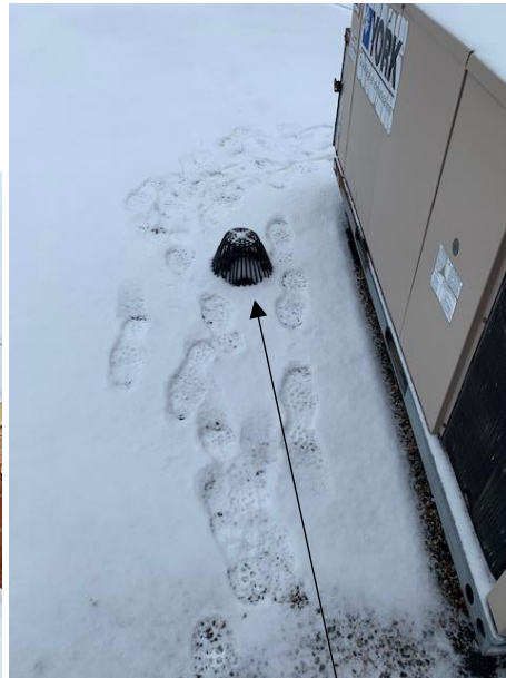
1 roof drain found near HVAC unit
