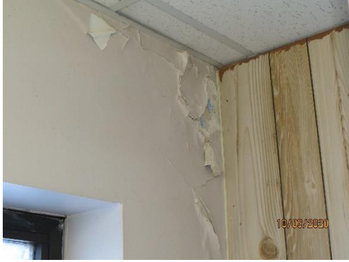
Upper floor bathroom
