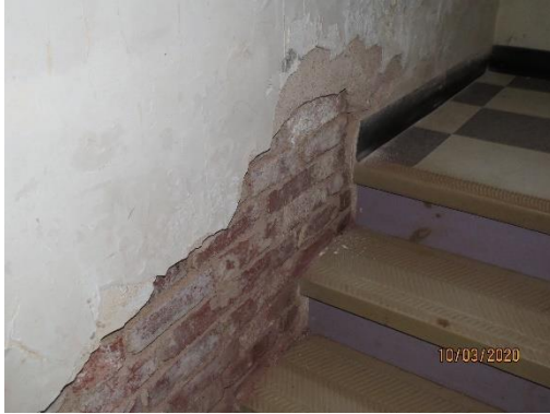
Stair to basement
