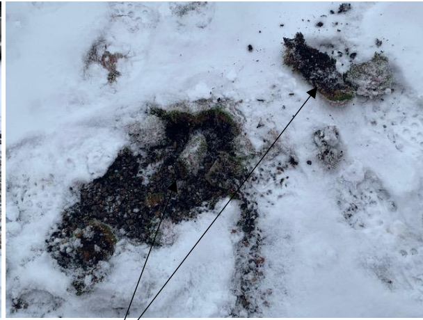
moss growth covered several areas
