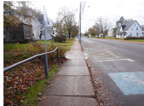
Accessible street parking spot outside of post office. Pavement is marked with horizontal signage (i.e., blue and white international symbol of accessibility). Side aisle is painted but uses existing driveway as curb ramp.
