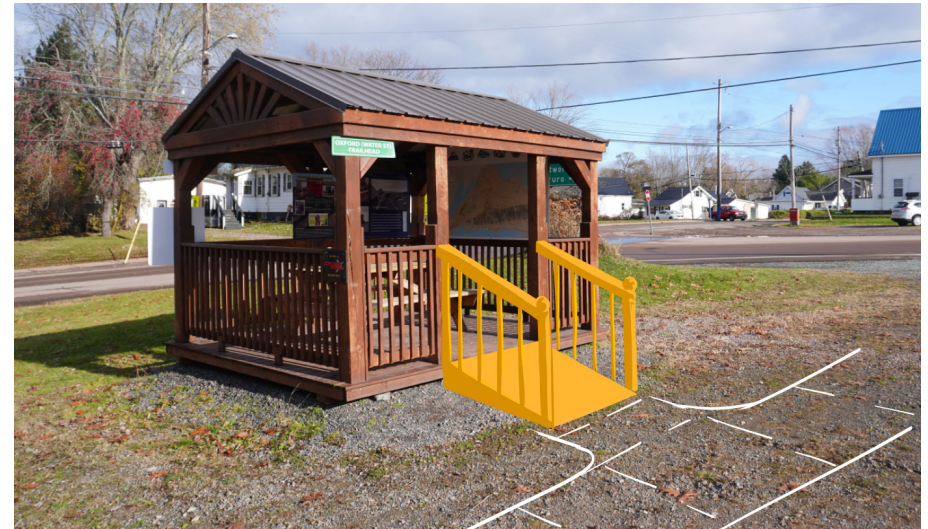
Figure 13. Example of an accessibility upgrade project. Ramp added to trails structure on Water St. at entrance to the Trans Canada Trail.
