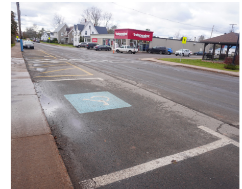
Accessible street parking spot on Main St. near pharmacy located on same side of street. No curb cut onto sidewalk from marked side aisle.
