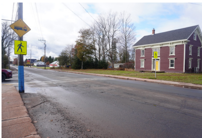
Yellow reflective signage on either end of Main St. crosswalk.
